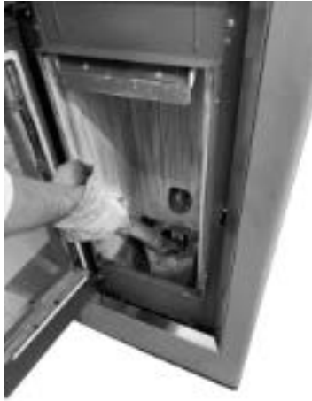
Fig. 35 - Burning pot box cleaning
